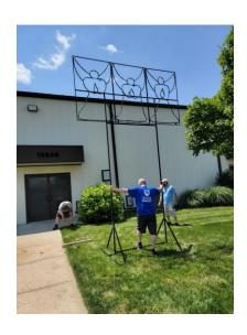
STEP 7: Provided with the Heavenly Host frame are Qty. 4 16' guide wires as well as stakes. Stake down the four guide wires (two in back, two in front) to support the display
